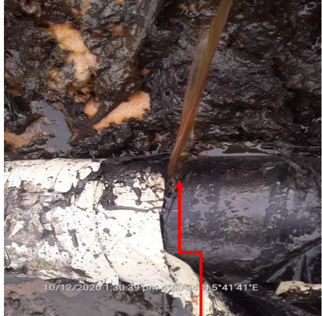
Fig B: Incident Facility shortly after excavation
