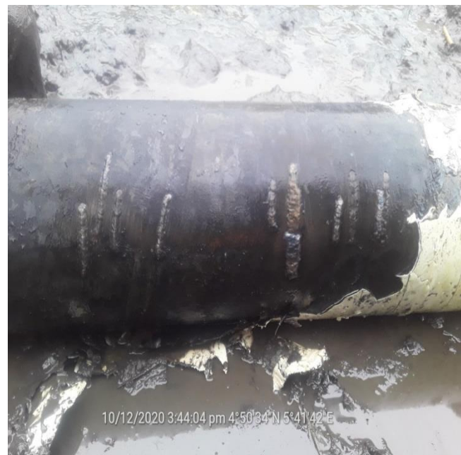
Fig D: Incident facility during repair
